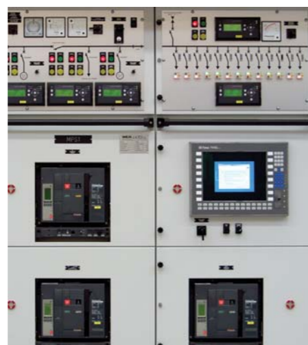
MILITARY SHIPS Man Machine Interface Groups management and control Fincantieri "HORIZON" Class Frigate
